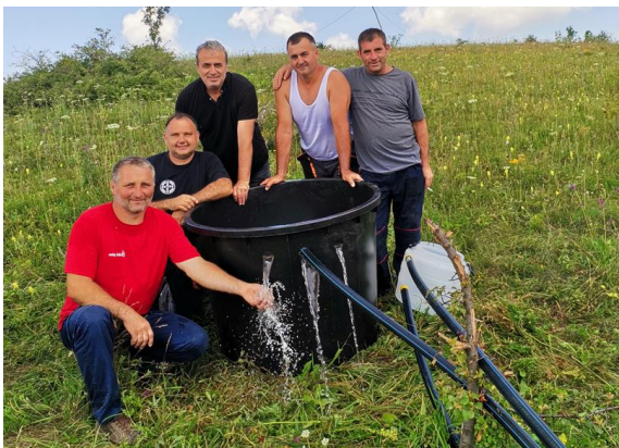
Picture 1: Installation of the irrigation system
