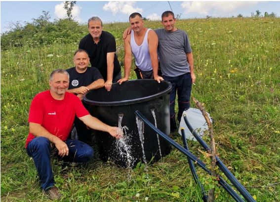
Picture 1: Installation of the irrigation system
